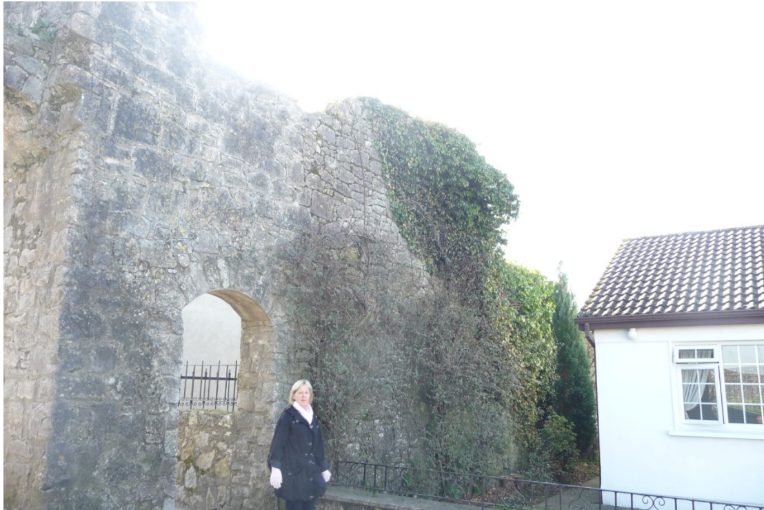
Pic 10: Wall West of North Gate Outside face.
