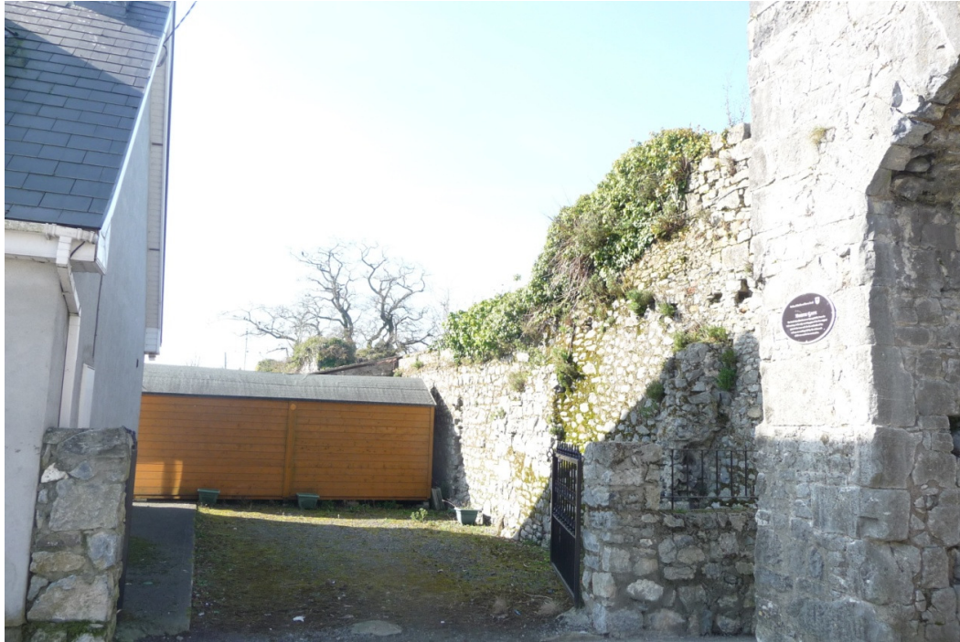
Pic 9: Wall West of North Gate Inside face.
