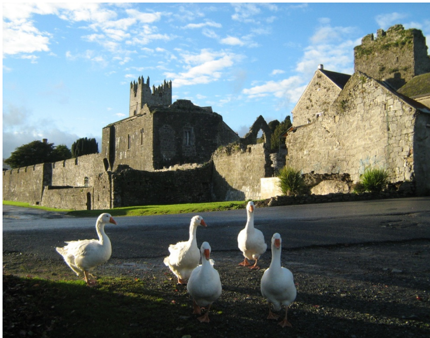
Pic 1: Repaired Section of Fethard Town Walls at Watergate, Fethard.
