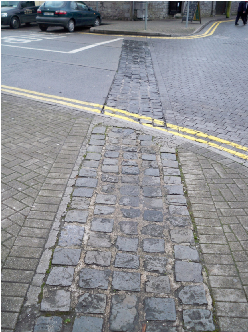
Pic 4: Example of wall marking in public street.
