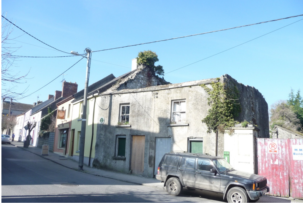
Pic 2: Façade and Wall Behind at Burke Street. Removal of façade will open town wall to public view.
