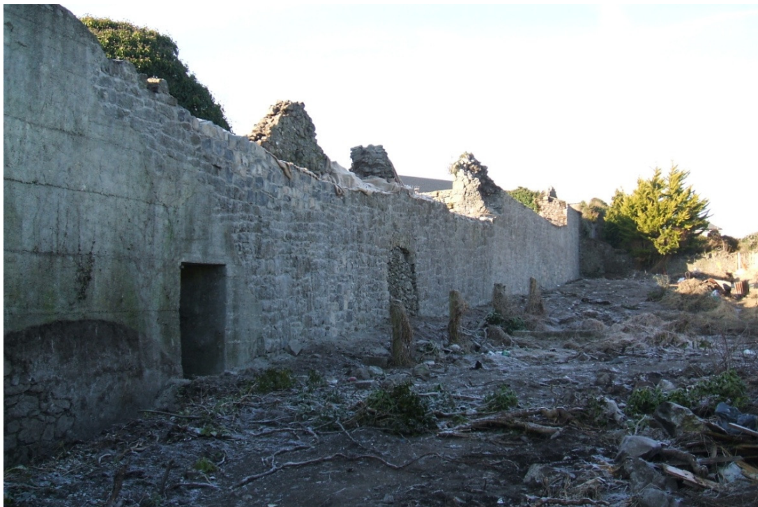
Pic 3: Wall hidden from view at Burke Street.
