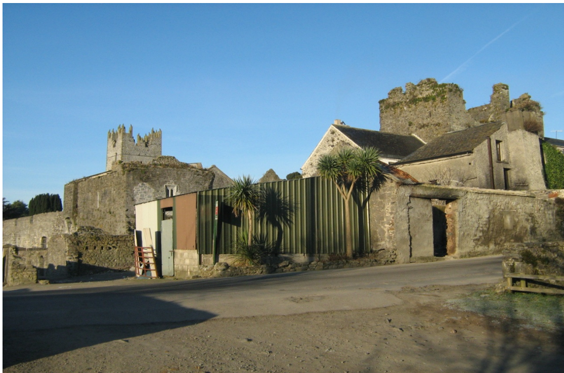
Pic 12. Showing site of wall Watergate with lean to structure obscuring town wall.
